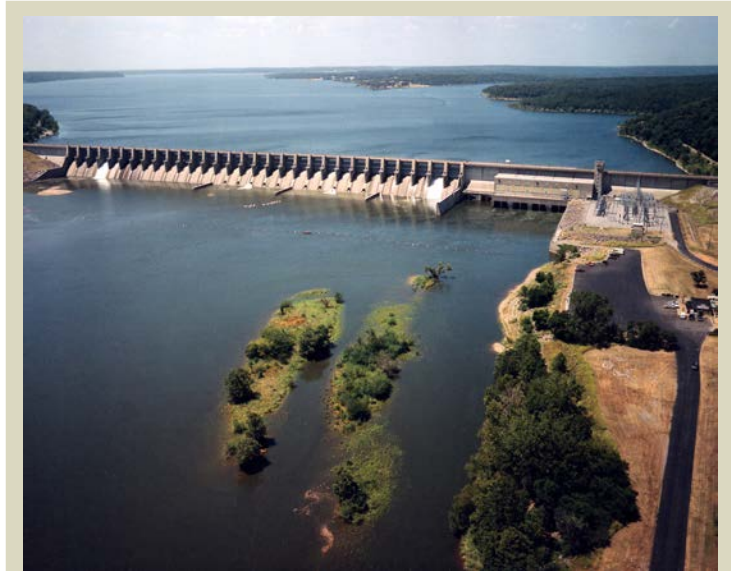
Fort Gibson Lake And Dam on the Grand (Neosho) River in Wagoner and Cherokee Counties. Construction began in 1941, and opened in 1946.
