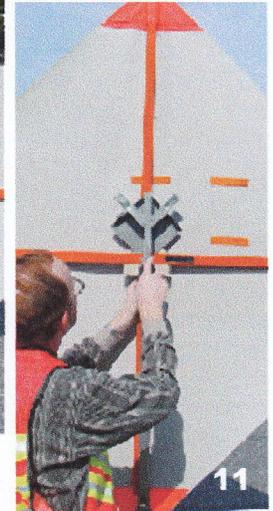
11. Raise the sign/Roll-up Sign Mounting Bracket so that the Horizontal Rib is the V-shaped Upper Sign Mounting Bracket and tighten the Screw Clamp of the Roll-up Bracket.
