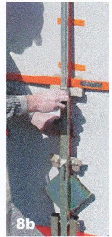
9. Raise the Mast/Sign assembly up until the bottom of the sign reaches the bottom of the lower Rigid Sign Mounting Bracket (the first snap lock for a 48" sign). Lock the Mast in that position using its Screw Clamp.
