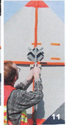
10. To mount a roll-up sign at the 60" height, leave the Roll-up Sign Mounting Bracket loose and place the Horizontal Rib behind and the Vertical Rib between the Ears of the Roll-up Sign Mounting Bracket.
