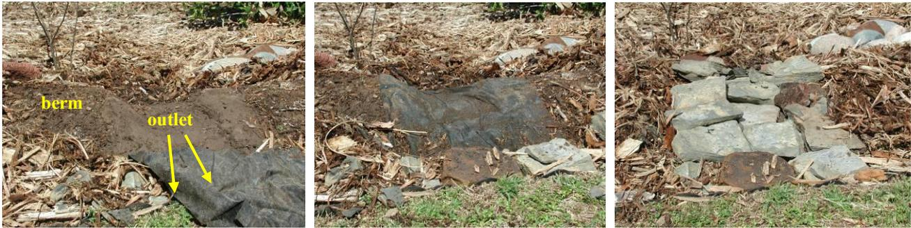
**Figure 2. Packed soil in the outlet notch in a berm (left). Proper covering of the outlet bottom, sides, and top (middle). Rocks covering the outlet (right). The berm keeps water in the newly developed rain garden. The outlet notch can be raised or lowered to ensure the rain garden retains the right amount of water.**
