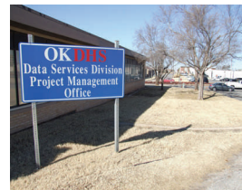
DHS/CAP BUILDING AT 50 N.E. 23RD ST OKLAHOMA CITY, OK
