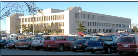
Department of Transportation Building Current Rating: 69 (+1)
