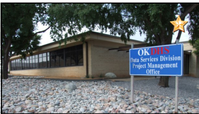
DHS-CAP Building Current Rating: 96 (E)
