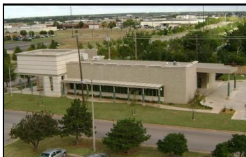
Banking Building Current Rating: 60 (E)
