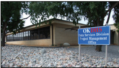
DHS-CAP Building Current Rating: 90 (N/A)
