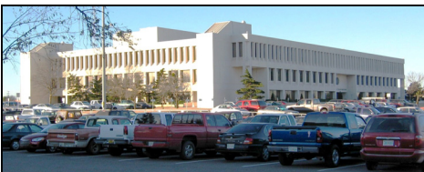
Department of Transportation Building Current Rating: 69
