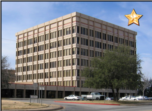
Kerr-Edmondson Building Current Rating: 89
