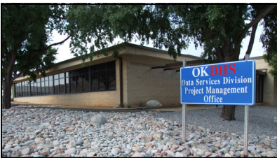
DHS-CAP Building Current Rating: N/A
