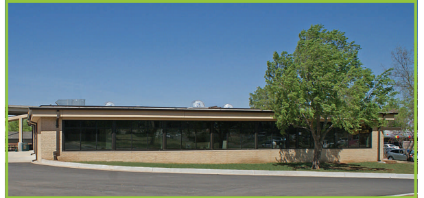
The CAP Building is located at 50 NE 23rd St. in Oklahoma City
