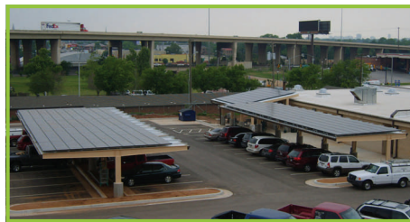
60 kW of PV solar panels on covered parking structures
