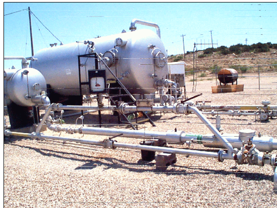
Figure 1. A test separator.
