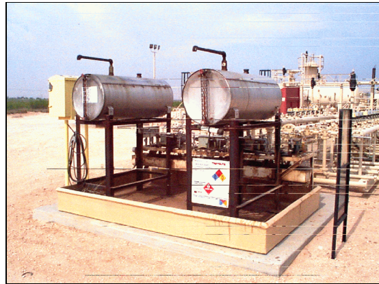
Figure 5. The chemical injection system for a large tank battery with injection at the header.
