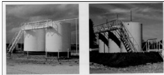
Figure 3. Examples of welded tanks (left) and fiberglass tanks (right).
