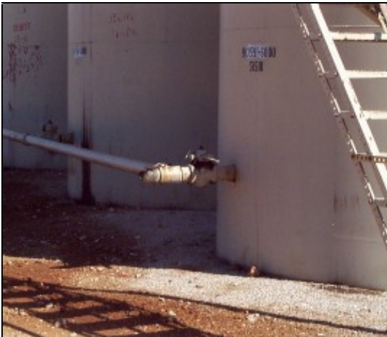
Figure 9. A Style 2 cone-bottomed tank showing how the sales outlet is raised above the BS&W level.
