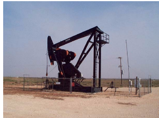
Figure 5. A security fence has been installed around this pumping unit because the well is near a busy highway.
