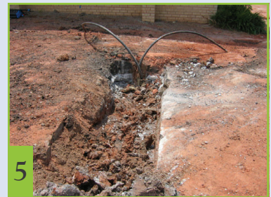
Geothermal well system fused together and ready to tie into building
