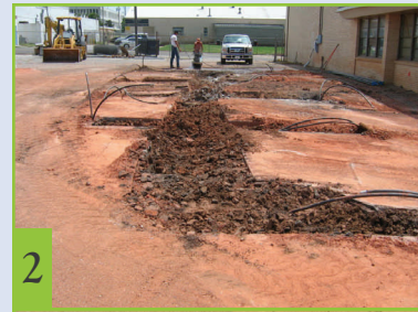
Beginning the process of digging out geothermal trench for piping
