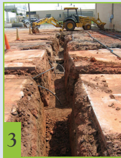
Trench dug to 4 foot depth
