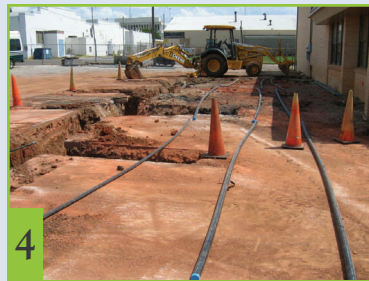
Piping laid out ready to be fused together and installed in trench
