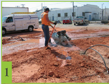
A worker cutting through concrete in order to dig geothermal trenches
