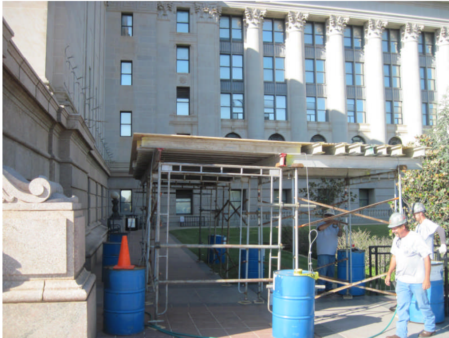
Photo 16 Debris Protection Scaffolding
