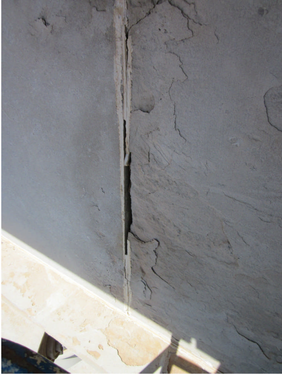
Photo 14 Southeast Corner: Deteriorated Mortar Joint Between Limestone Blocks, Spalling of Limestone Block Face, Spalling at Limestone Ledge
