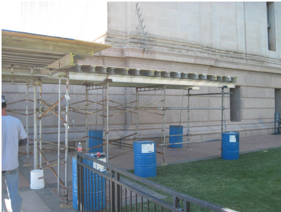
Photo 17 Debris Protection Scaffolding
