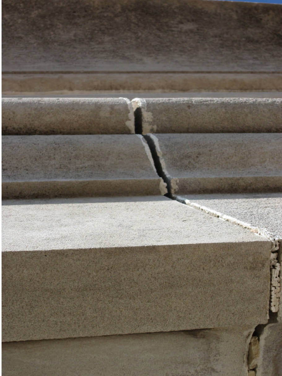
Photo 11 Southwest Corner: Deteriorated Mortar Joint Between Limestone Cornice Pieces
