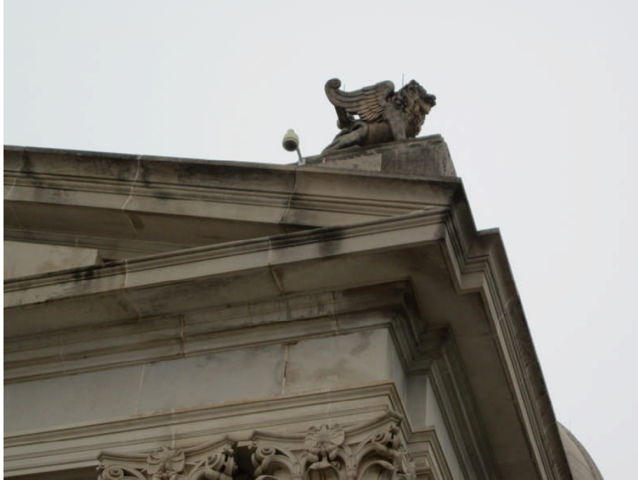
Photo 5 East Corner of South Portico
