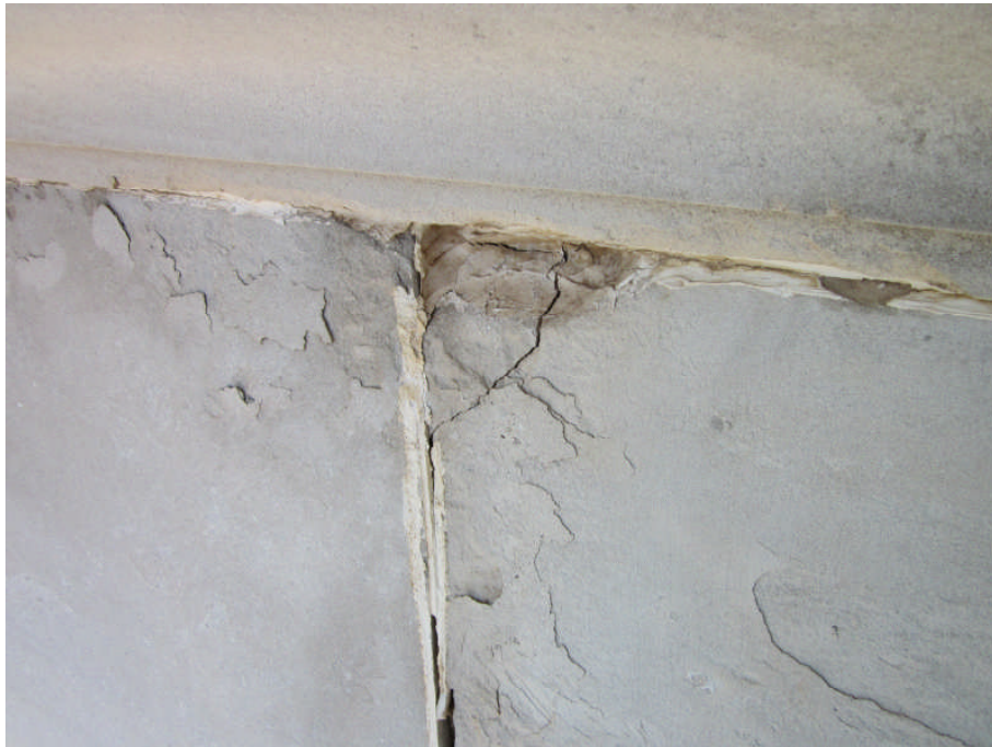
Photo 13 Southeast Corner: Patched Broken Limestone Block Corner
