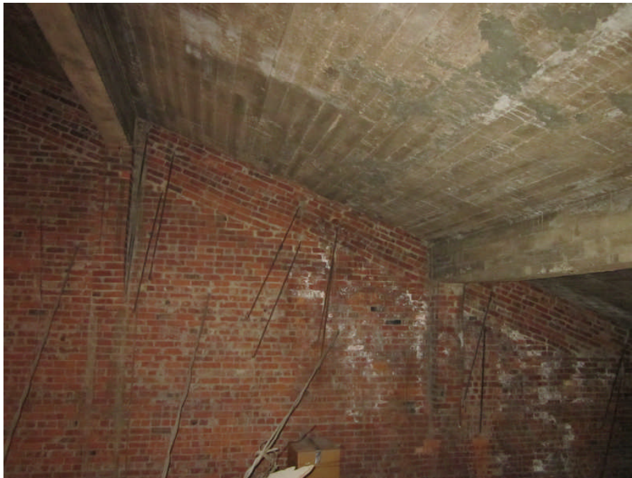
Photo 2 Concrete Roof and Beams with Clay Brick Infill
