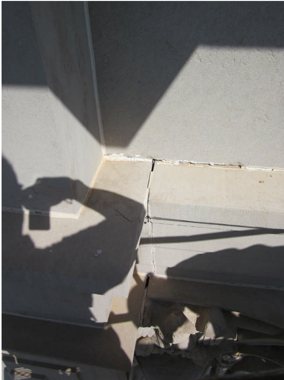
Photo 12 Southwest Corner: Deteriorated Mortar Joints in Limestone Ledge
