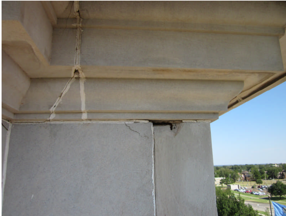
Photo 7 Southwest Corner: Broken Limestone Corner and Exposed and Corroded Steel Tie
