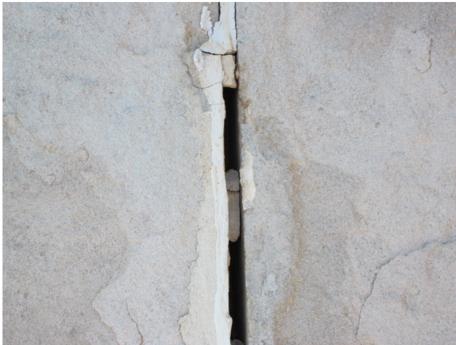
Photo 10 Southwest Corner: Deteriorated Mortar Joint Between Limestone Blocks
