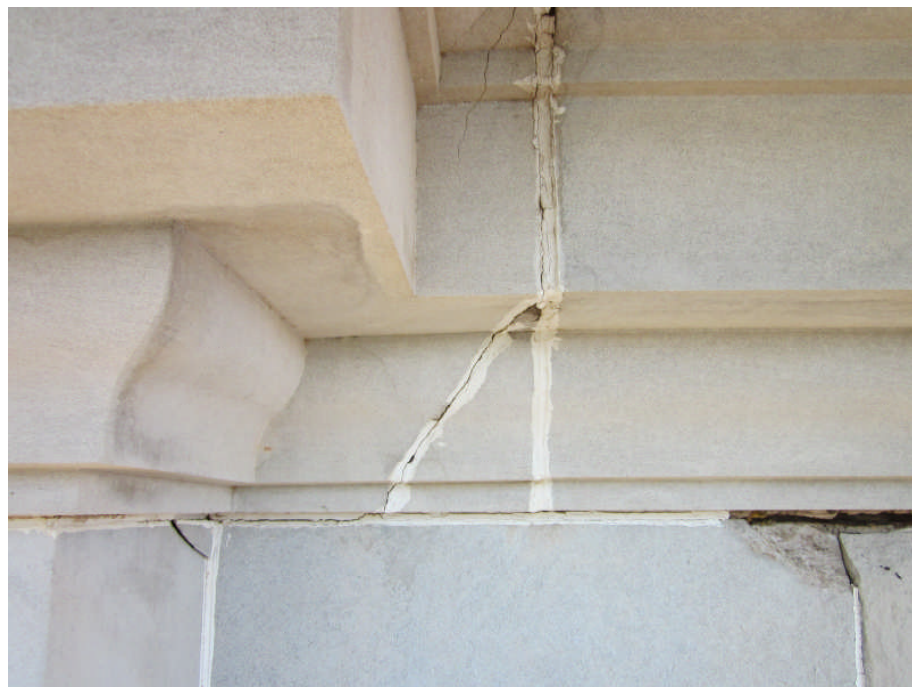
Photos 8 Southwest Corner: Deteriorated Mortar Joints, Crack Limestone Block Corners, Exposed and Corroded Steel Tie
