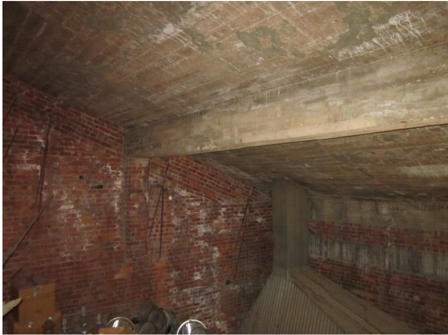
Photo 3 Concrete Roof and Beams with Clay Brick Infill
