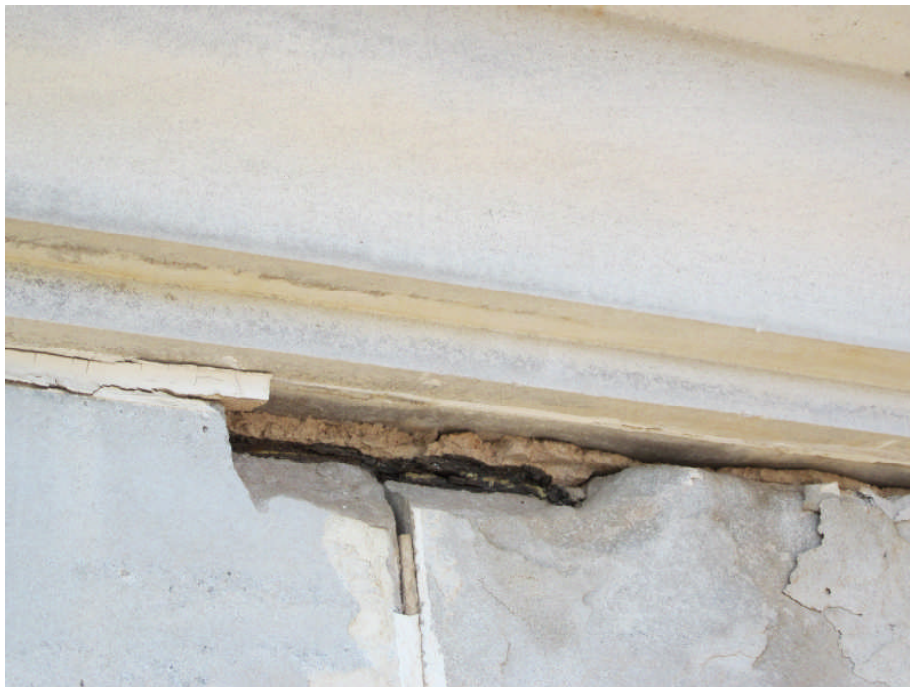
Photo 6 Southwest Corner: Corroded Steel Tie at Upper Corners of Limestone Blocks
