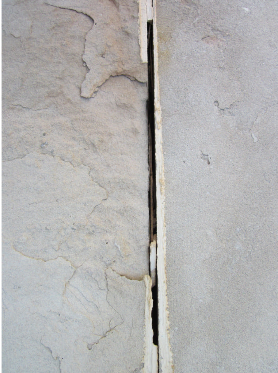
Photo 15 Southeast Corner: Deteriorated Mortar Joint and Spalling Face of Limestone Block
