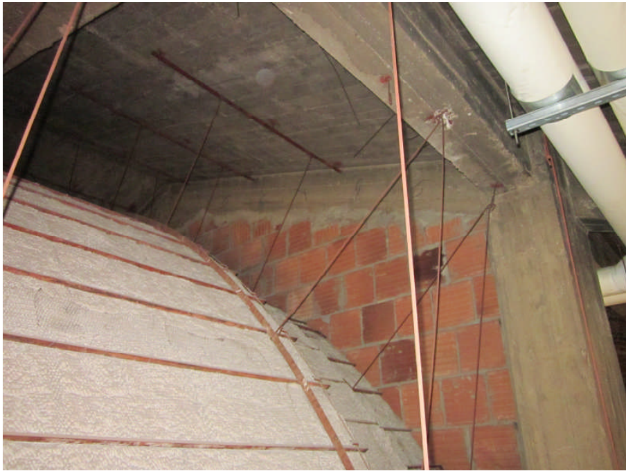
Photo 1 Concrete Frame with Clay Tile Infill
