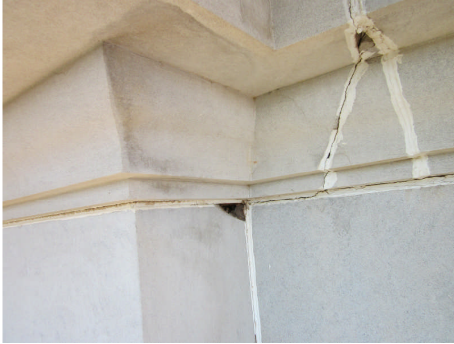
Photo 9 Southwest Corner: Deteriorated Mortar Joints and Crack Limestone Block Corners
