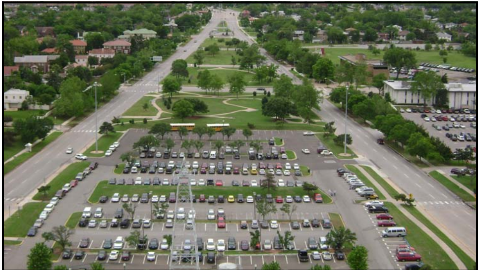
View of South Capitol Plaza where funds from the ODOT tree grant will be applied.
